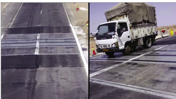
Figure 2: The WIM technology is composed of two platforms
