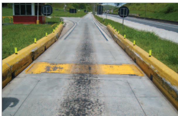
Figure 7 Detail of fixed scales in the weighing station
