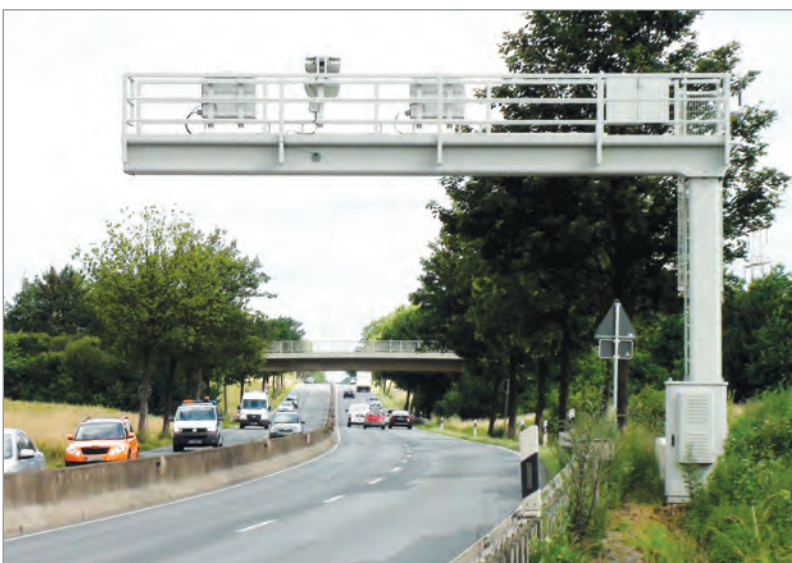
Figure 1: Entrance portal of the first ASC in Germany. The gantry houses the lane cameras for vehicle identification and the laser scanners for triggering.
